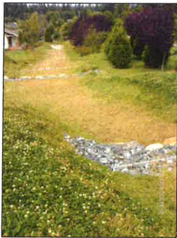
SILVER BEACH CREEK BIOINFILTRATION SWALE
