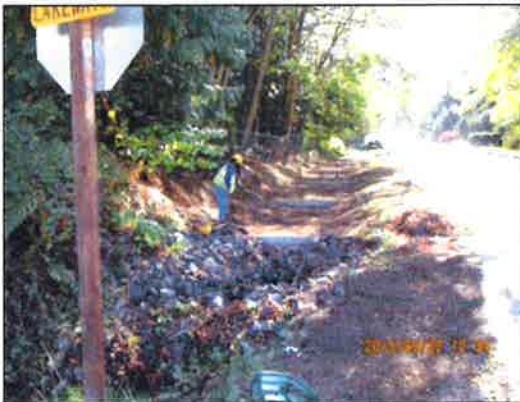
BIOINFILTRATION SWALE REPAIR AND ENHANCEMENT AT LAKEWOOD LANE AND LAKEWAY DRIVE (BEHIND GENEVA ELEMENTARY SCHOOL)
