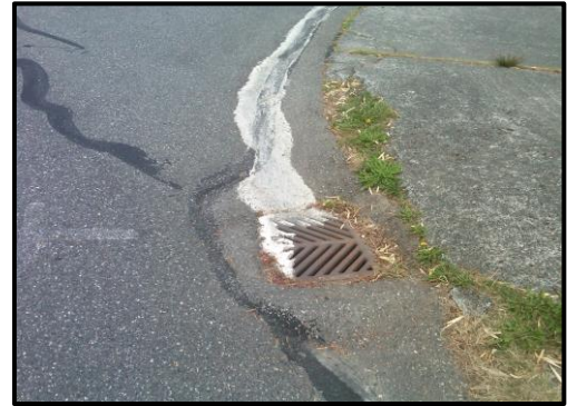
Soapy water entering catch basin
