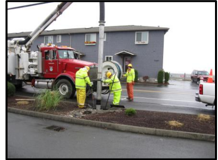
Catch Basin Cleaning in Birch Bay
