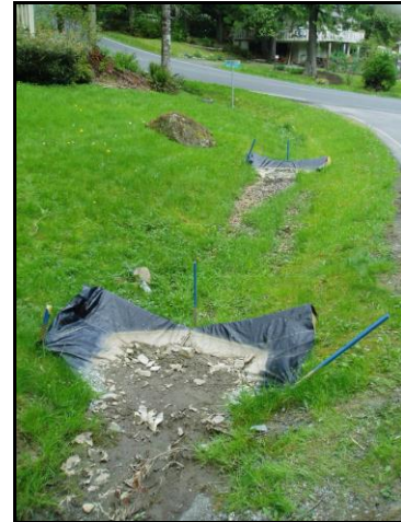
Triangular Silt Dike
