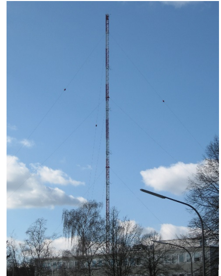
Figure 1. Typical Meteorological Tower
