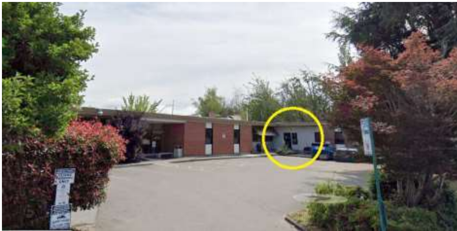
View of 509 Girard Street from the Grand Avenue Parking Lot
