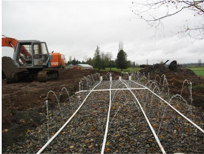
If the pump tank is pumping the sewage to an above ground sand mound, then the system type is a **Pressure Mound**. A pressure mound has all the same components as a pressure distribution system except for the drainfield.
