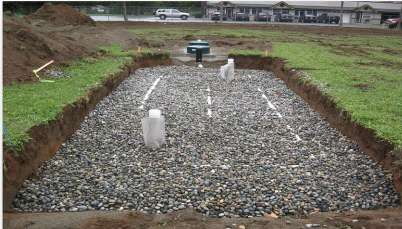
Due to differences in elevations, on some occasions, a pump is needed to get the sewage to the drainfield. Once the sewage is at the drainfield, it is dispersed via gravity within the drainfield. Examples of these types of systems would be a **Pump to Gravity Distribution** or a **Non-Pressurized Mound** (Gravity Mound).
