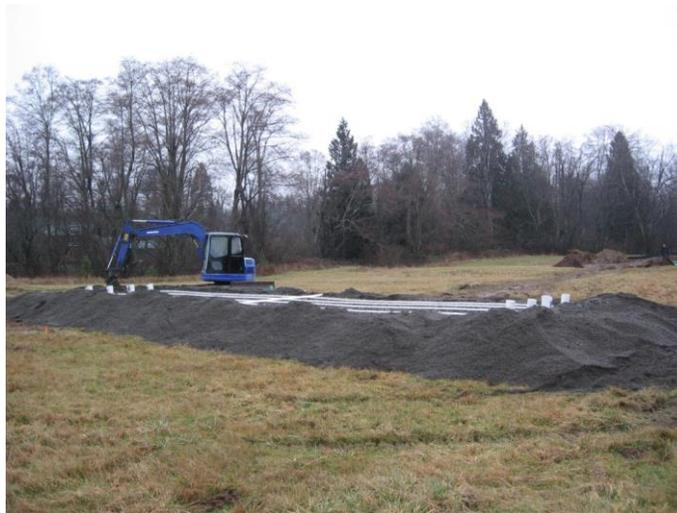
Sometimes prior to the drainfield (gravity or pressure), the sewage may pass through a **Sand Filter**. A sand filter can be constructed of either a flexible membrane or a concrete vessel. In a sand filter, the sewage is distributed evenly throughout the vessel and then it passes through several feet of sand and gravel, providing additional treatment of the waste. The sewage is then captured after the sand filter and distributed to a drainfield.
